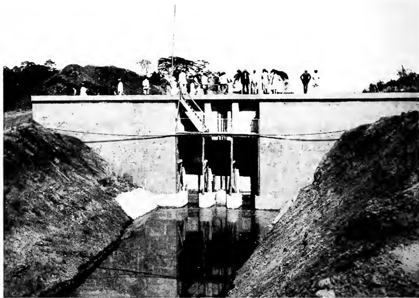
GUAYUBÍN IRRIGATION CANAL View of the principal sluice gate
